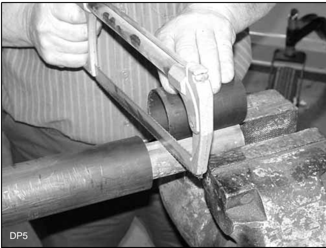
Figure 9. Cut Shaft to Length
